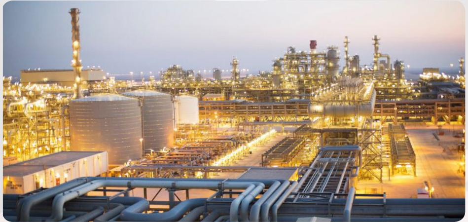
The Pearl GTL Plant is capable of producing 140,000 barrels of GTL product each day. The plant also produces 120,000 barrels per day of natural gas liquids and ethane.
